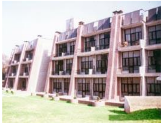
South view of building showing solar water heating panels and solar chimney
